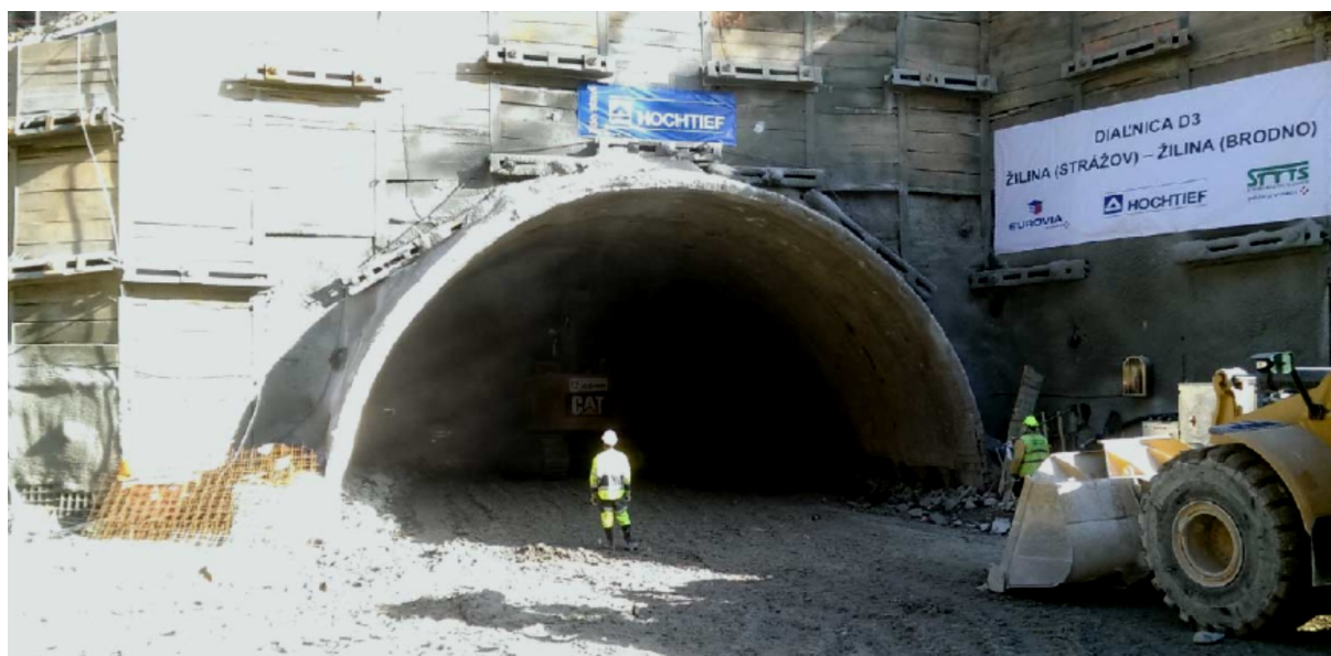
Figure 6: Central part of tunnel – view on east portal.
