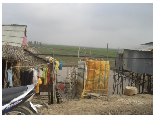
Fig. 1 – A toilet on a ditch – a common type in rural areas in the Mekong Delta
