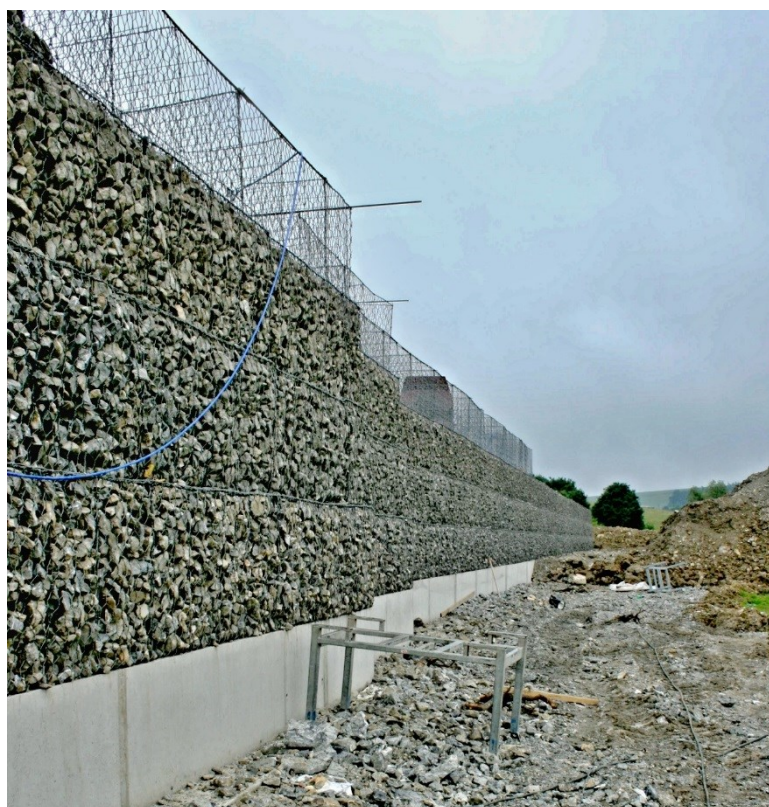
Figure 1. Construction process of gabion wall
