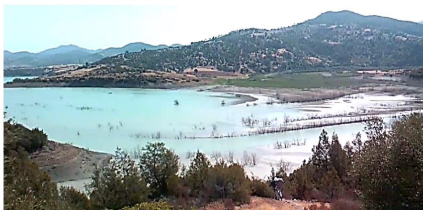
Figure 5. Vase deposit upstream of the Oued Fodda dam (Photo: Benkaci, August 2017)
