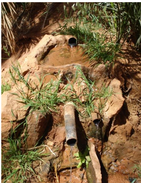
Figure 15. In the oasis of Timimoun, a kasria unrecognizable due to PVC (Photo: Remini, 2008)
