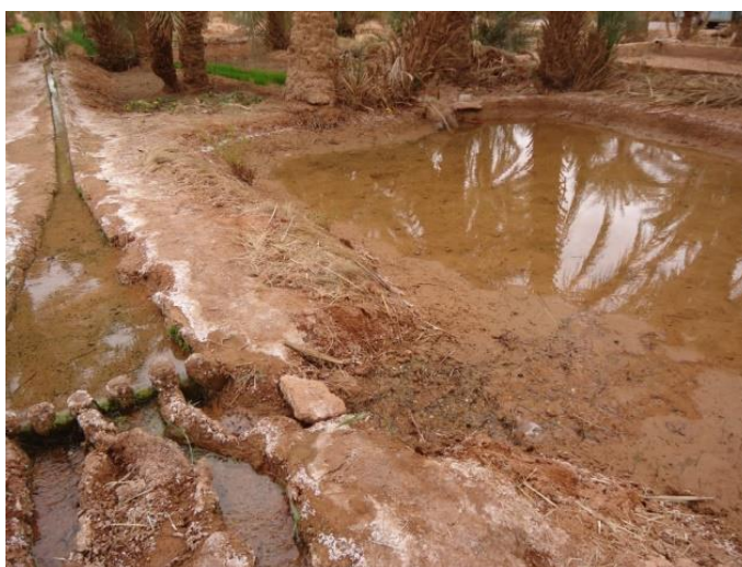
Figure 5. Madjen and secondary Kasria of an In Ghar Foggara in the Tidikelt region (Photo: Ghachi and Remini, 2013)
