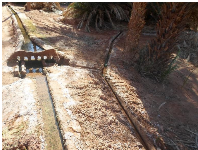
Figure 4. Secondary Kasria of an In Ghar Foggara in the Tidikelt region (Photo: Ghachi and Remini, 2013)
