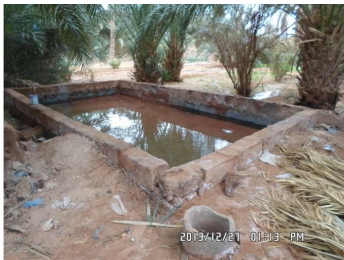
Figure 10. Madjen realized in cement in the palm grove of Irsan (Photo: Ghachi and Remini, 2008)
