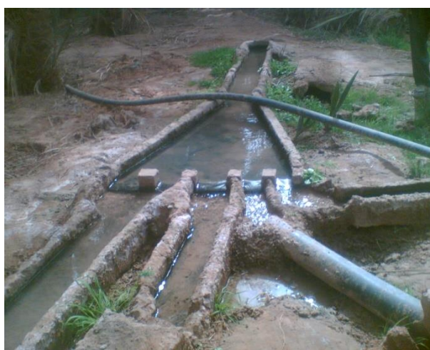
Figure 14. Even the Kasriates have been modified by the addition of PVC pipes (Photo: Ghachi and Remini, 2013)
