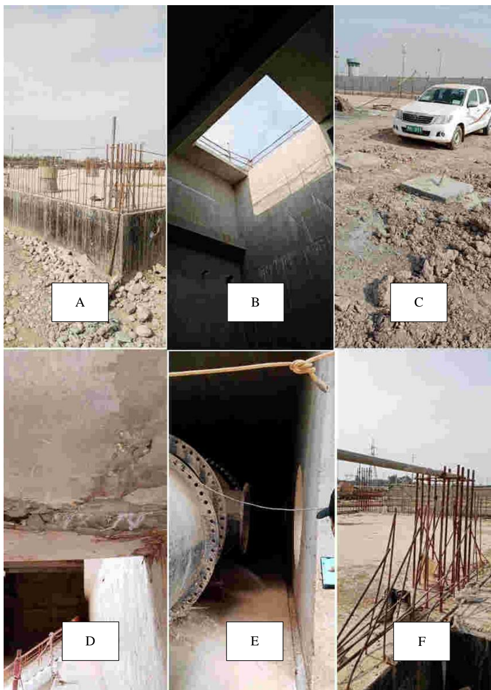
Figure 2. Pumping station after being exposed to the subsidence due to water withdrawal outside the station and below the foundations. A) The outside view of the pumping station site; B) The inner side view of the pumping station; C) The withdrawal of water below the foundations of the pumping station; D) Fractures in the skeleton of the pumping station; E) Pipes damaged due to soil subsidence; F) Joints due to soil subsidence (Photo: Al-saady, 2020)
