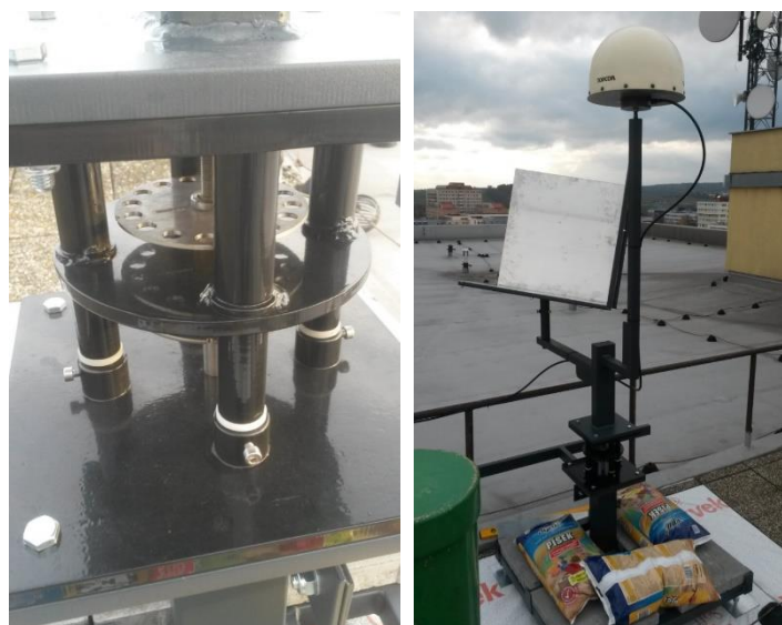
Figure 3. Detail of a produced adjustable device (left) and an overall look on a whole construction containing adjustable device, corner reflector and GNSS antenna (right)
